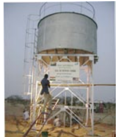
The first bore-hole finishing construction.
